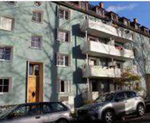
Figure 7.8.3: Balcony Additions done in unison to entire building
