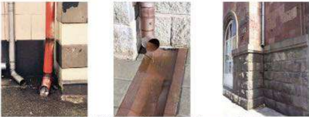
Figure 7.12.4: Trench Drain represented above are not allowed.
