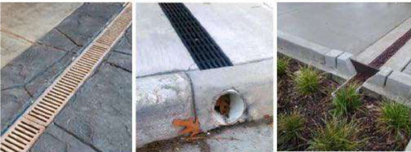
Figure 7.12.5: Trench Drain represented above are allowed.
