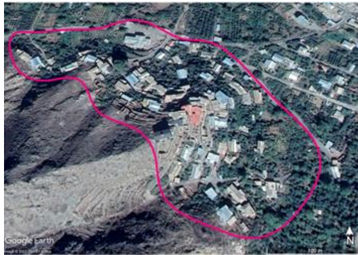
FIGURE 1: STUDY AREA BOUNDARIES. PROPOSED CORE AREA EXTENDING OF A SURFACE OF 13.5 HA AND FOCUSING ON POQR TAGH DISTRICT
